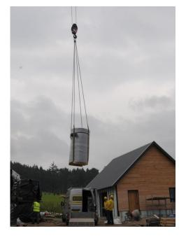
The SOLARFOCUS Therminator II 40kW boiler has an integral fueling chamber that is 186 litres and a rated output of 36kW when running on logs. The boiler is connected to a 2000 litre thermal store which allows the thermal store to hold approximately 70kWhrs of energy every firing. The boiler is also capable of running automatically on pellets via a vacuum system and Schellinger Pellet Mole.
